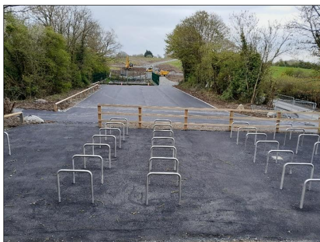
Parking Area – Countryside Park
