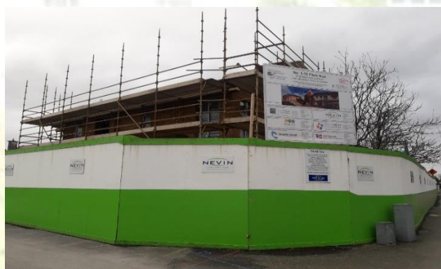
Construction Works at Pairc Nua [Broguemaker], Castlecomer Road
