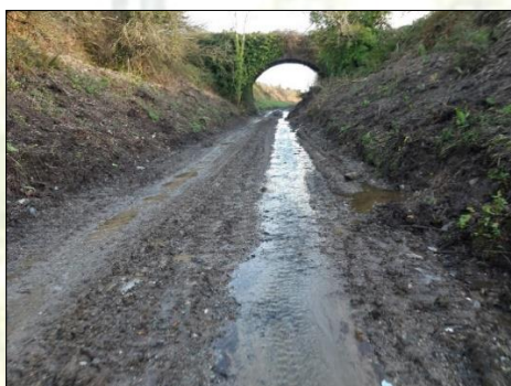
December 2020 - View of old railway track through the Ferrybank urban area
