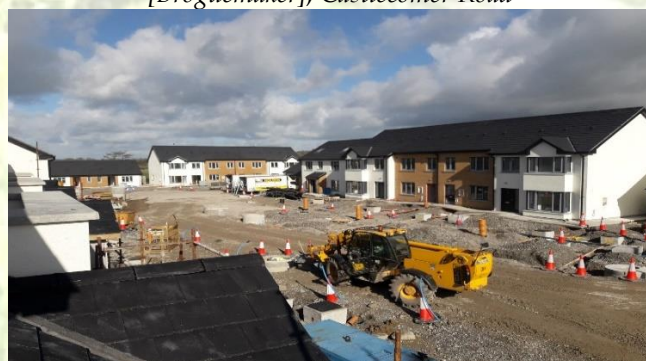
Construction Works at Station Avenue, Ballyragget
