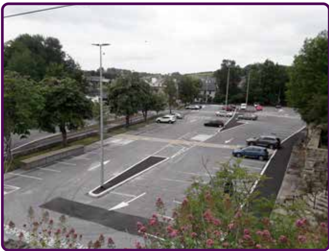
The Quay Carpark Thomastown
