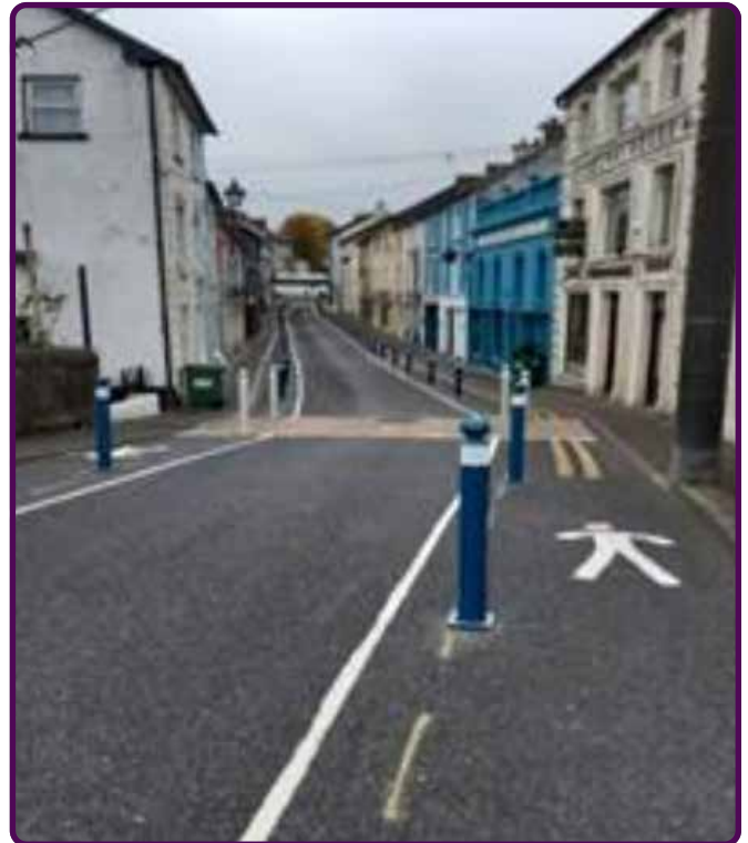
Provision of extra walking space at Bridge Street, Callan
