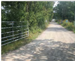
6 MAIN PATH - 3M WIDE COMPACTED LIMESTONE DUST
