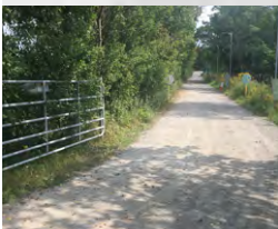
6 MAIN PATH - 3M WIDE COMPACTED LIMESTONE DUST
