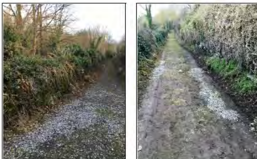
Figure 2.3 Simple grass verge and roadway maintenance to L66013
