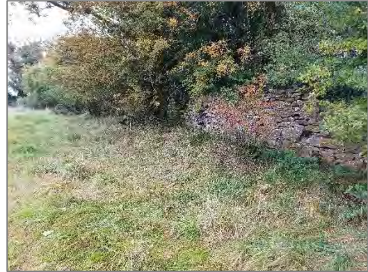
Stone wall viewed from southern side
