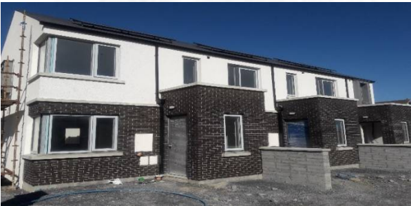
38 units under construction at Hoban Park, Callan
