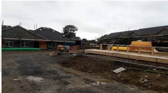
17 Units at Breagh Place, Main Street, Piltown
