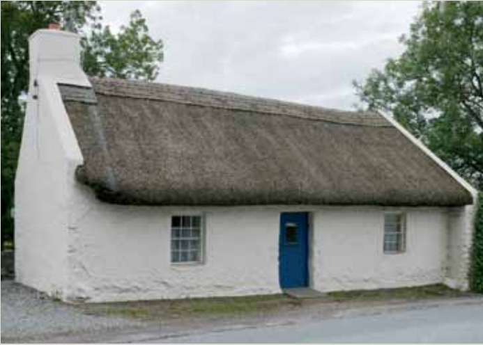
A roof in County Cork with raised gable copings to protect the edge of the thatch from wind uplift. These gable copings also cover the edge of the thatch as can be seen at the eaves detail
