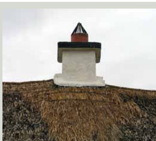
Typical rendered masonry chimney with mortar flaunching at the base and firmly scoloped thatch around it
