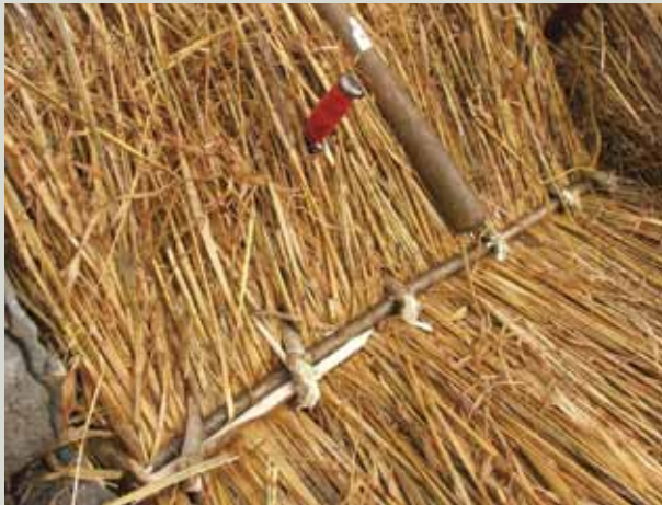
A course of thatch is fixed firmly in position with a scollop keeper and several hairpin scollops
