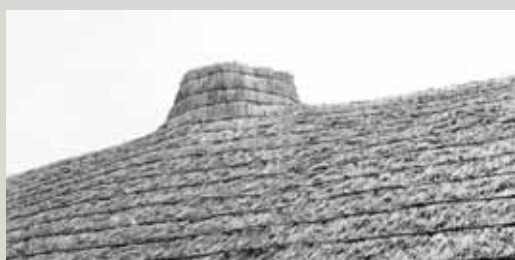
Thatched chimney, County Clare. Caoimhín Ó Danachair (Image from the National Folklore Collection, University College Dublin)
