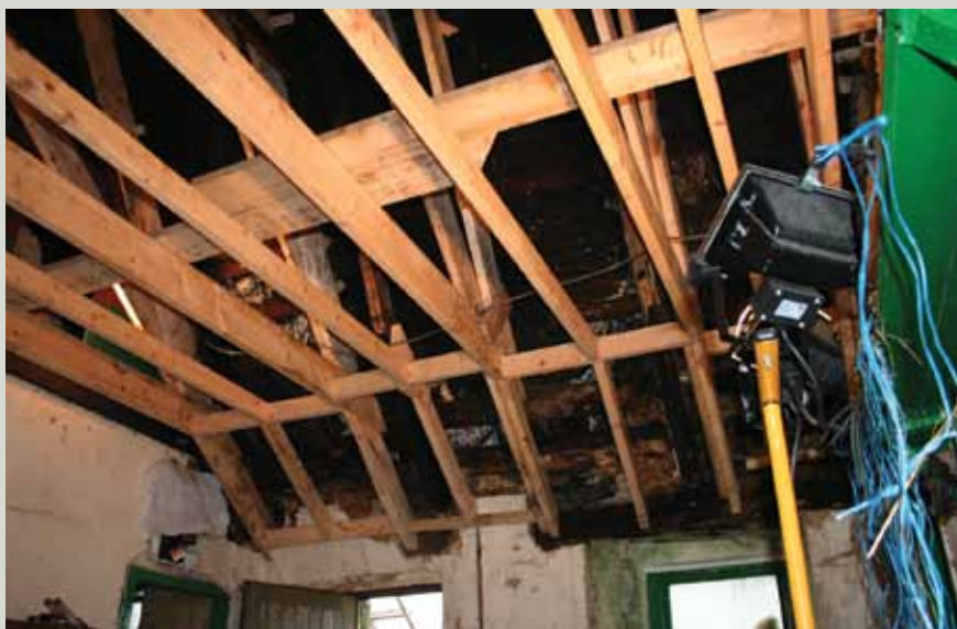
A new roof structure has been inserted beneath an old roof, strengthening and, at the same time reinforcing, the original structure which has been left in place above. However, a major intervention of this type is only justifiable where there has been a widespread failure of the existing structural elements
