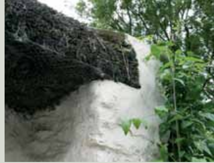
A roof in County Cork with raised gable copings to protect the edge of the thatch from wind uplift. These gable copings also cover the edge of the thatch as can be seen at the eaves detail
