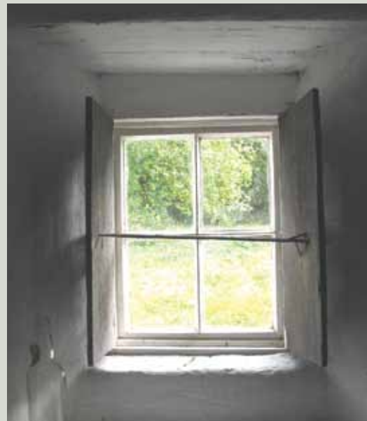
A small sash window with simple internal shutters is typical of vernacular houses
