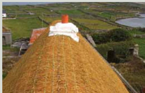
Roped thatch with flush (rounded) ridge
