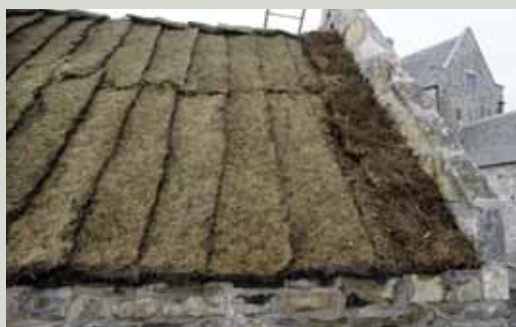
Scraw laid on a reconstructed roof
