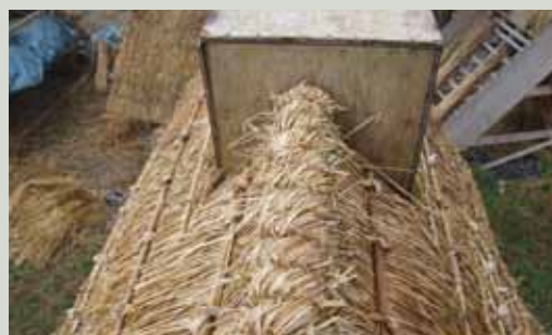
Straw flush ridge with bobbins and rodding (Image courtesy of Brian Simpson)
