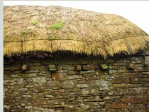
An example of roped thatch in County Donegal. Ropes passed over the roof at regular intervals secure the thatch against high winds and are tied to stones projecting from the walls
