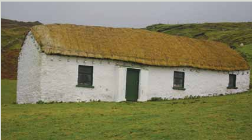
An example of roped thatch from County Donegal – a method of construction developed in response to the high winds experienced along the exposed Atlantic coast
