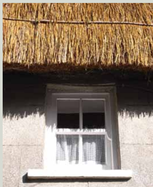
Straw thatch, in County Wexford, using horizontal stretchers to pin and tighten the eaves
