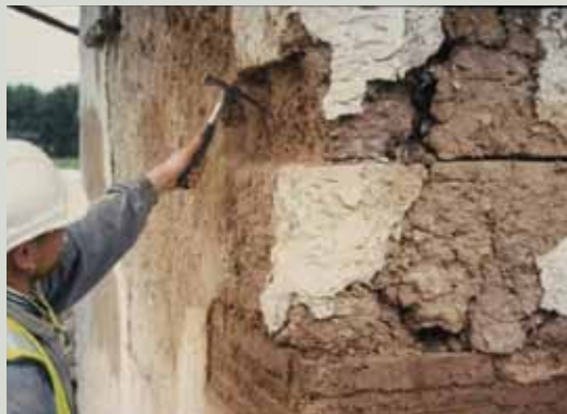
Repair of a corner crack in an earth wall
