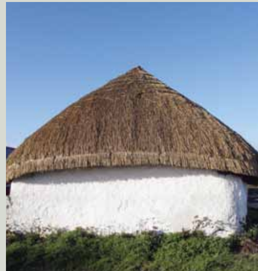
A hipped roof of oat straw thatch on an earth walled house in County Offaly
