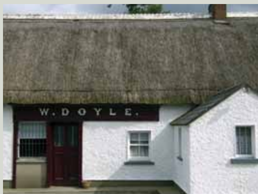
Thatched roofs in parts of Leinster were sometimes finished with decorative external ridge boards such as this example from County Wexford
