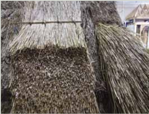
An exhibition of contrasting methods of thatching – showing scolloped rye thatch to the left and thrust wheat straw thatch on the right (Image courtesy of Brian Simpson)
