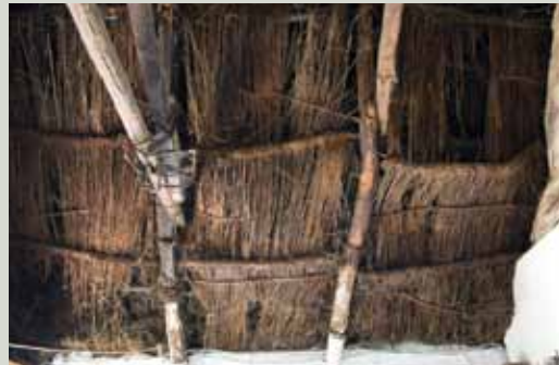
Straw lining to the underside of a roof in County Limerick
