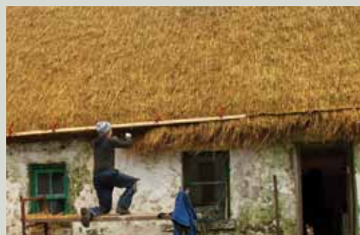
Trimming the eaves following a re-thatch
