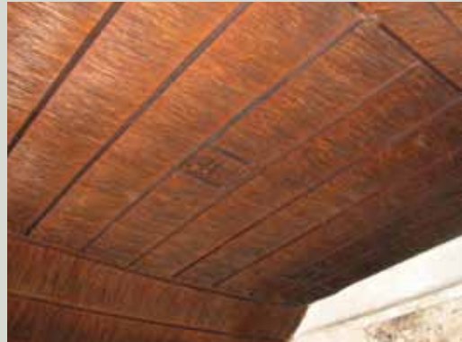
Ceiling made from reed fleeking
