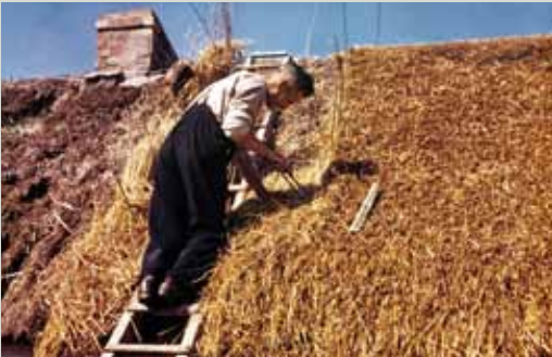
Thatcher driving home a hairpin scollop. Caoimhín Ó Danachair (Image from the National Folklore Collection, University College Dublin)
