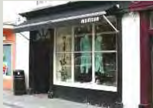
A new awning has been successfully fitted to this shopfront without the need for a visually obtrusive blind box
