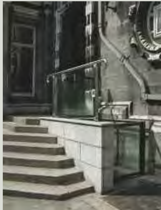
A well-designed platform lift of a sympathetic design using high quality materials, and provided in addition to, and not as a replacement for, steps may be acceptable. However, alternative solutions may have to be explored where a symmetrical or harmonious composition would be unbalanced or damaged by the addition of a ramp
