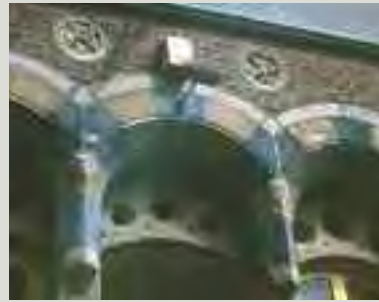
Inappropriate grit-blasting or chemical cleaning methods may ultimately shorten the life of stonework by removing the protective skin of the stone, exposing it to greater environmental damage, or may damage the appearance of the stonework by blurring arrises, tooling or carved work, as has happened in this example
