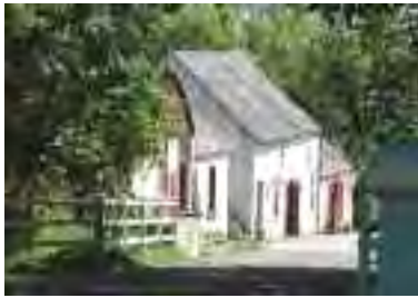
In rural areas, former settlements or groups of buildings can survive substantially intact thus adding to the special historical interest of the area
