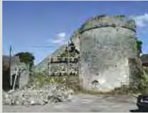
Ivy has been removed from this mediaeval mural tower after an detailed record was made of the fabric to ensure that potential loss or damage to the stonework could accurately be remedied, reusing the historic fabric without resort to conjecture
