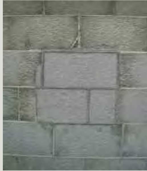
The repair of concrete structures should be carried out so as to resolve the underlying problem without a visually obtrusive result. In this illustration the repair to the reconstituted 'stone' will tone down in time although the strap repointing is inappropriate
