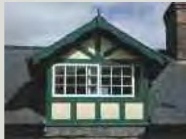
Original dormer windows were usually designed as part of the architectural vocabulary of a structure and may contain a wealth of detail such as finials, ridge tiles, bargeboards and slate-hung or glazed cheeks
