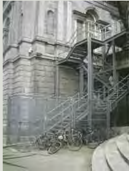
The use of external escape stairs should be avoided on important elevations or where they would be obtrusive in an important view of the structure
