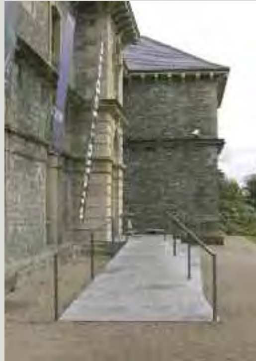
Modern interventions can be acceptable where they use high-quality design and materials. Such work can address the needs of the users while respecting the architectural quality of the structure
