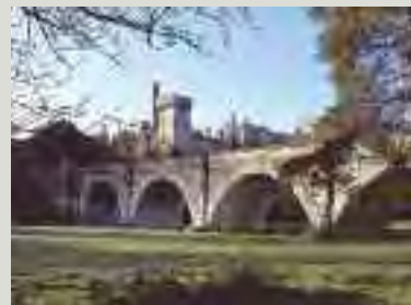
Some protected structures such as bridges, follies and other iconic landmarks are strong, self-contained compositions that may be difficult to alter without affecting their character and special interest
