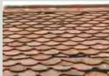
Clay roof tiles, though widely used in other countries, in Ireland rarely date from before the latter half of the nineteenth century. Either flat or profiled (pantiles) they can be decoratively shaped, as in this instance
