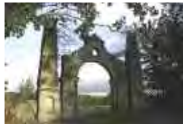
Protection can extend to features within the attendant grounds of a protected structure provided they are specified in the RPS. Alternatively they can have a separate listing in their own right
