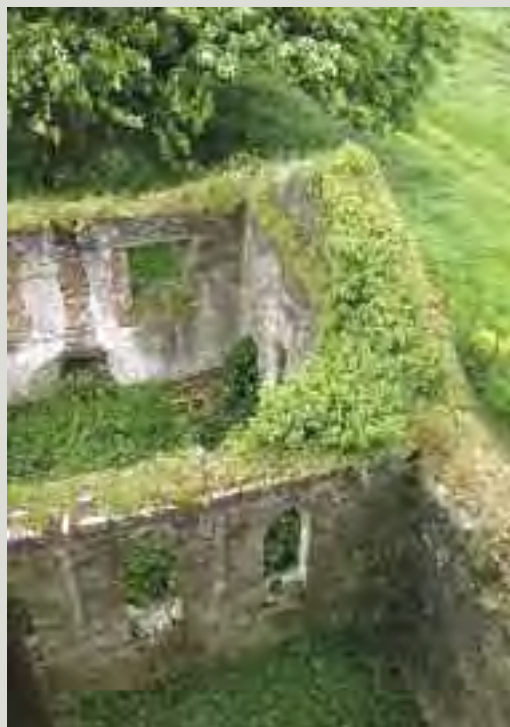
Exposed wall heads are generally the most vulnerable parts of a ruined structure. The method proposed to cap exposed wall heads should not result in water being trapped inside the core of the wall and should be visually acceptable. In some cases, the ruinous structure may need to be monitored over a period of time before a decision can be made as to what work might be appropriate
