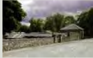
The style and materials of structures used to demarcate the boundaries of a protected structure, its curtilage and attendant grounds can add significantly to its character and that of the surrounding area. This rubble stone wall and fine stone gate piers line the approach to an important complex of stables and farm buildings
