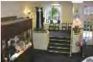
The careful removal of later alterations of little interest, such as this half floor and steps, may be exempted by a declaration
