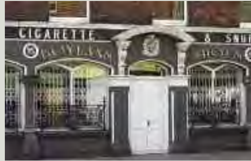
Where good lettering or signage exists but a premises has changed hands, it may be possible to add new signage while leaving the original lettering in place. For example, a new signboard can be mounted over the existing one without damaging the original lettering below or, as in this illustration, new signage can be placed elsewhere on the shopfront, leaving the old name in place
