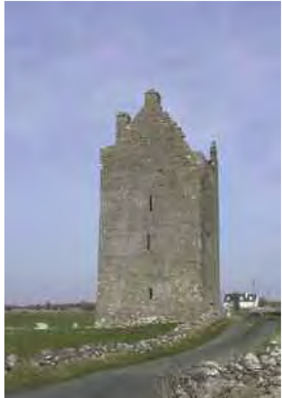
Many structures are of both architectural and archaeological interest and suitable for protection under the Planning Acts in addition to the National Monuments Acts
