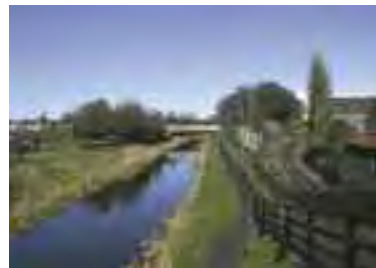
The special technical interest of an area may derive from its association with industrial heritage areas or landscapes such as harbours, ports, railways and canals
