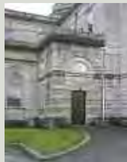
The option of re-grading the ground adjacent to an entrance could be considered where the difference in levels is small, where the raised level would not conceal architectural details, where there is no loss of historic pavement and of course where sufficient ground is available to create a gentle gradient
