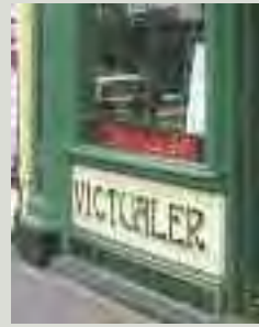
The functional and decorative features common to many historic shopfronts including tiled stall risers (top), ornate brackets (middle) or original shutters (bottom) are all part of the special interest of a shopfront
