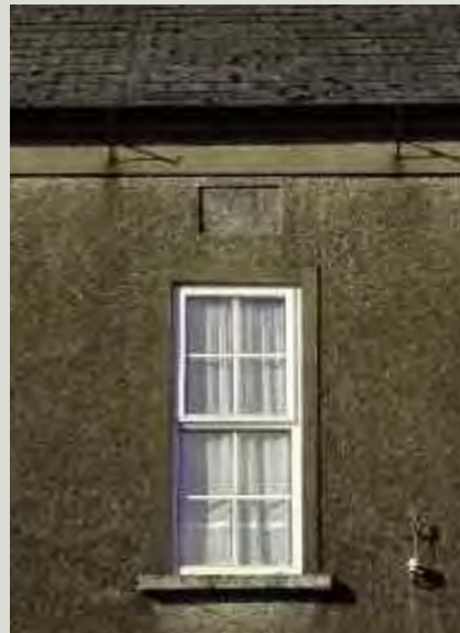
Over-restoration or poorly specified replacement elements can be as much a threat to the character of historic structures as neglect or wilful damage. In this case, the datestone of 1736 is one of the few surviving original features on the exterior of this house
