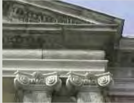
The application of proprietary spikes or wiring may be necessary to deter birds congregating as their droppings damage masonry. Such additions to architecturally significant buildings should be designed to be unobtrusive and reversible
