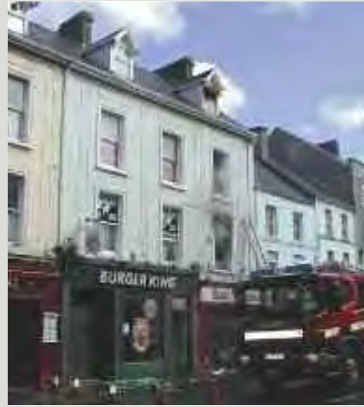
Many fires are successfully extinguished before major damage occurs, requiring a careful assessment of the remaining fabric to ascertain if its special interest has been compromised. An assessment of the extent of reinstatement appropriate following partial damage will require to be carried out on a case-by-case basis
