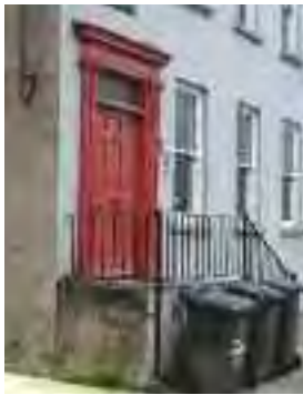
Consideration should be given to the storage of waste disposal bins as these can have a large visual impact on an area
