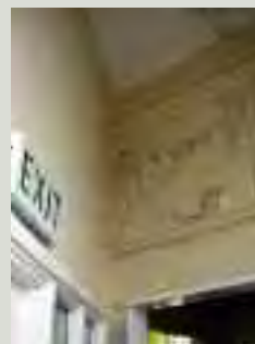
The design of a new protected lobby within a fine historic interior should take great care to avoid adverse visual and physical impacts; interrupting a symmetrical space or cutting across decorative plasterwork may not be acceptable regardless of whether the proposed works are reversible
