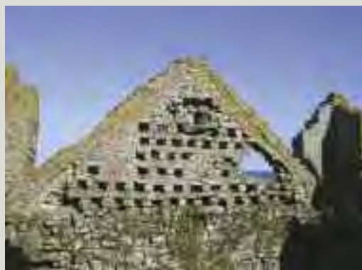
Some ruins may require careful dismantling and re-erection of parts of walls that have become unstable. In this case, apart from the repair work required to the gable (containing pigeon nesting boxes), it is intended to re-roof the building. Where it is appropriate to re-roof a ruinous structure, the aim should be to retain the maximum amount of original fabric
