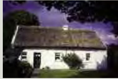
Irish vernacular thatching is simple in its construction and detailing, addressing, in the choice of roof profile, structure, materials and weathering details, the prevailing climatic conditions and available materials
