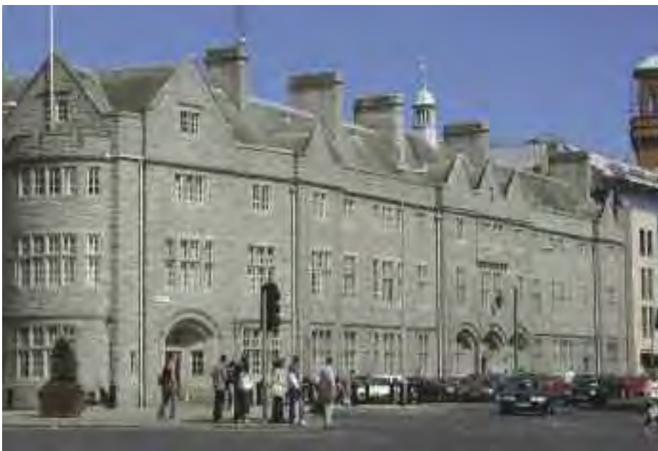
Certain building types such as Garda Stations, subject to the provisions of Part 9, are also protected structures
