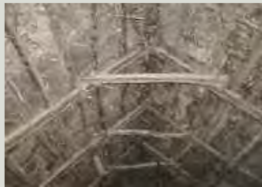
Unwrought or partially-wrought roof structures, however simple or slight they may seem, are part of the historic vernacular fabric. Repairs should aim to support the existing structural elements with new timbers rather than replace them
