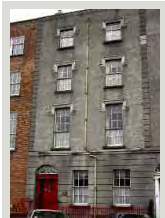
Alterations of different periods may contribute to a knowledge and appreciation of the history of a structure. The application of plaster hood-mouldings to earlier buildings was fashionable at the end of the nineteenth century. While they may now appear anachronistic, they can also be seen as part of the unique history of that building
