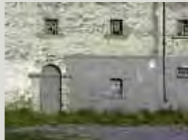
The conversion of this 1762 Charter School nursery to a store in the nineteenth century involved partially blocking the window openings, thereby altering its character. Restoring the openings would be possible using surviving evidence in the fabric and employing historically accurate detailing. This approach is appropriate where the character of an architectural composition can be restored by undoing later alterations of little interest
