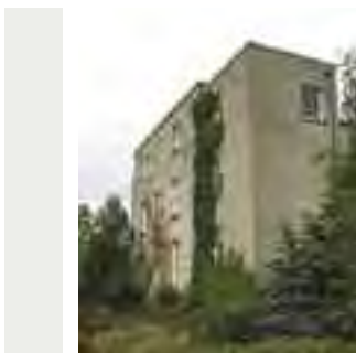
Later extensions of little interest can be carefully demolished without adverse impact on the protected structure as with this later stair tower added to the rear of an eighteenth-century villa
