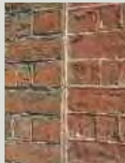
Inappropriate grit-blasting or chemical cleaning methods may ultimately shorten the life of stonework by removing the protective skin of the stone, exposing it to greater environmental damage, or may damage the appearance of the stonework by blurring arrises, tooling or carved work, as has happened in this example
