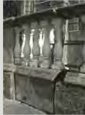
This elaborate access gate to the basement area is fabricated of plate and cast iron to match the adjacent stone balustrade. Surviving high-quality eighteenth-century iron balustrading such as this is rare and significant
