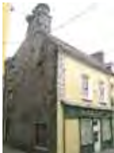
Upstanding structures protected under the National Monuments Acts can be considered for inclusion in the RPS such as this building which contains a substantial amount of mediaeval fabric
