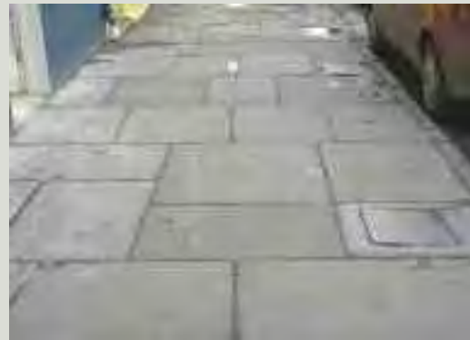
While coal holes are often considered part of the public domain, they may in fact be part of a protected structure whose cellars extend below the pavement, in this case one paved with fine flagstones. There are regional and local variations to the design and shape of coal hole covers, many impressed with their manufacturers' names
